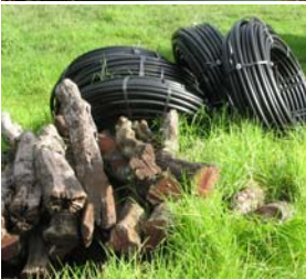
2,000 feet of water pipe & Kiawe wood railings are ready for installation.
