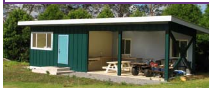
Shed is complete with 2011 plans for an 800 square foot covered area workshop extending off front of building.
